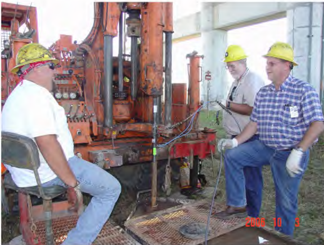
Fig. C-6 CME-750 All Terrain Rig with Instrumented Rod and Automatic Hammer Attached
