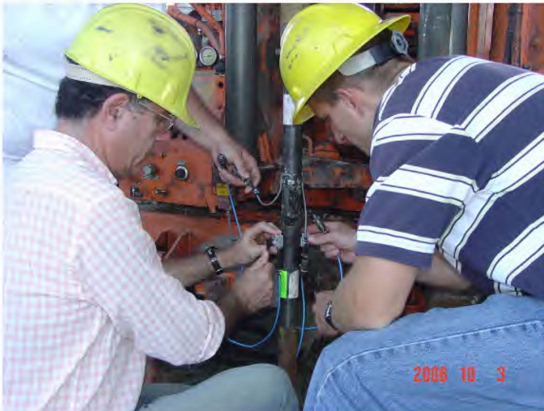
Fig. C-4 Mounting Accelerometers on Instrumented Rod
