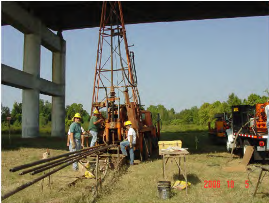
Fig. C-3 Failing 1500 w/ Dietrich Hammer Drilling at Primary Test Site
